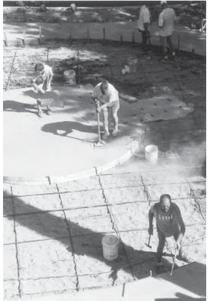
Before the concrete hardened, a design was stamped into the surface to give it an old world texture.
