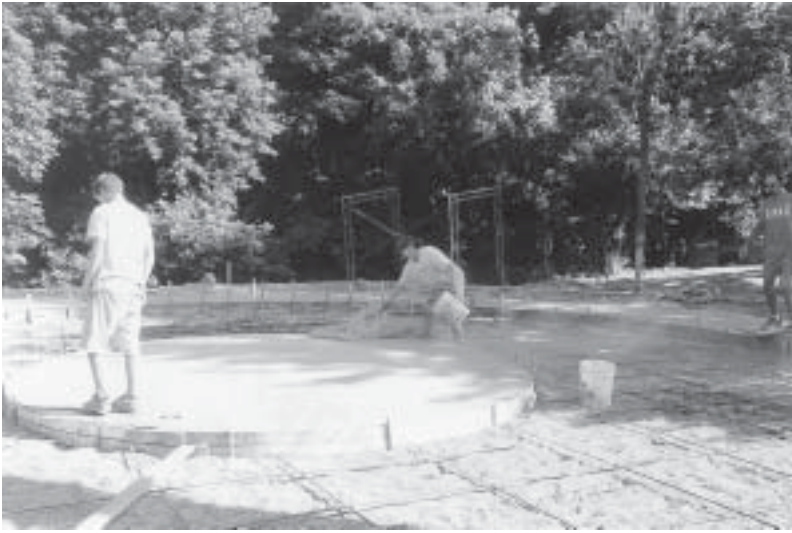
Craftsmen spread three subtle colors of powder into the setting concrete to make the surface more interesting.
