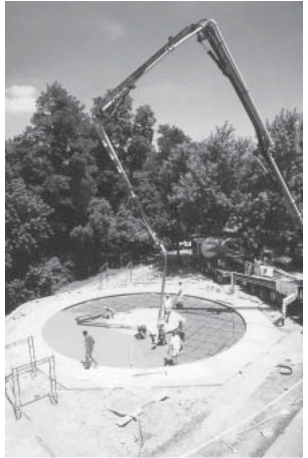
Swackhammer Masonry & Concrete pours concrete into the design forms in late July.
