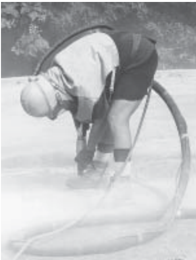
Craftsmen spread three subtle colors of powder into the setting concrete to make the surface more interesting.
