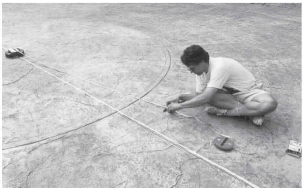
Before the concrete hardened, a design was stamped into the surface to give it an old world texture.
