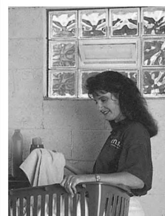
Replacement Basement Windows Installed With Air Vents
