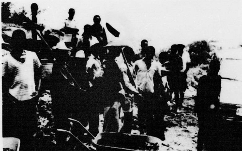
DREAM ROAD —Men are "hand-building" a road near Les Orangers, Haiti, to replace a rugged path. The pastor of St. Matthew's adopted parish there wants the road for access to the medical, educational, material and spiritual needs of his people.
