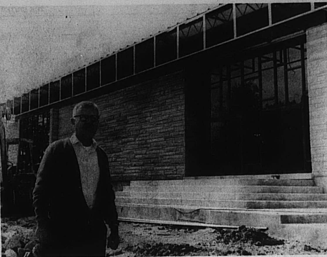
SELLERSBURG CHURCH NEARS COMPLETION—Father Aloysius A. Barthel, pastor of St. Paul's parish, Sellersburg, is shown in front of the nearly-completed new parish church. Parishioners expect to be attending Mass
