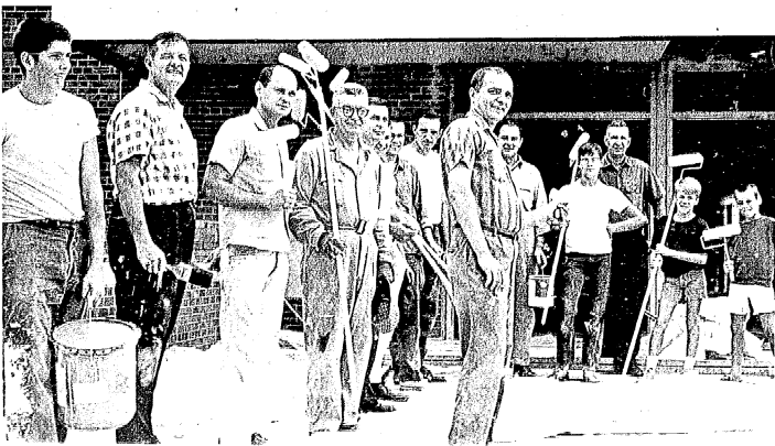
NEW SCHOOL PAINTED BY VOLUNTEERS—One of the many projects being handled by laymen on the new Pope John XXIII Grade School, in Madison, is the painting of 24,000 square feet of concrete block walls and partitions. Nearly 50 men and boys have devoted recent week-ends to the project, which has required 450 gallons of paint. Other major activities being handled by laymen include the seeding and fertilizing of the lawn, installation of driveways, clock and sound systems and kitchen equipment. The new 16-classroom consolidated school will serve four parishes in the Madison area, replacing existing facilities at St. Mary and Mt. Calvary schools in Madison. Occupancy is planned for November 1. It is located adjacent to Shaw Memorial High School.
