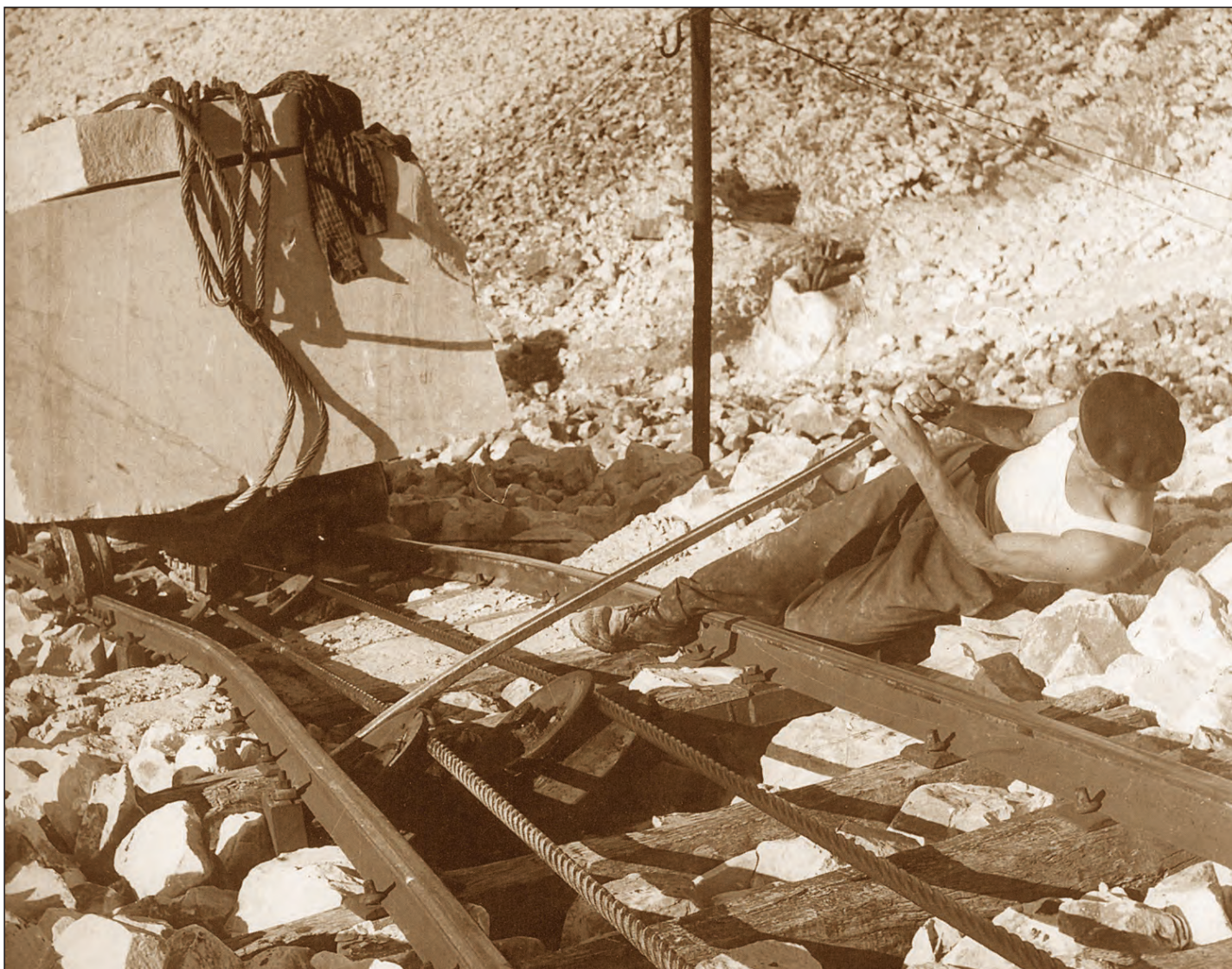
Stonecutters move blocks of marble that weigh as much as 40 tons from the quarries in Carrara, Italy, with lizzatura , pieces of wood laid on the slope so heavy ropes could be used to ease the cut stone down the mountain. A dozen men hold the ropes for resistance while other men manage the ropes on the descent, letting gravity do as much of the work as possible.
