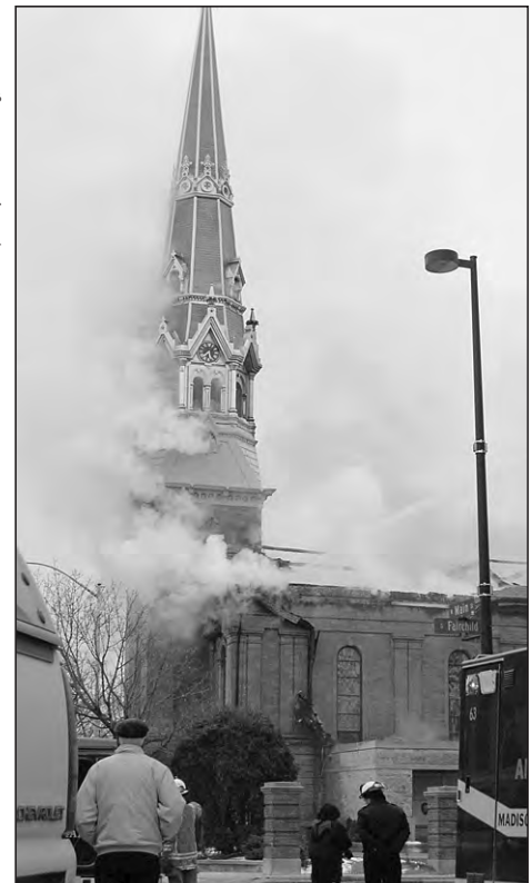
Cathedral rector Msgr. Paul J. Swain, left, watches as smoke billows from the steeple and roof of the 150-year-old St. Raphael Cathedral in downtown Madison, Wis., on March 14. The early morning fire destroyed the roof of the cathedral and caused significant damage to the interior. No injuries were reported from the fire. The cause was unknown.
