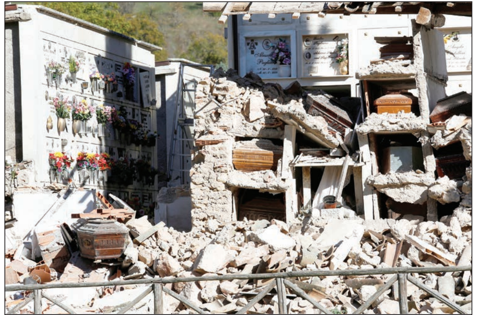
Coffins are seen in a collapsed cemetery on Oct. 31 following an earthquake near Norcia, Italy. Priests in central Italy were instructed to celebrate Mass outdoors following another devastating earthquake that rocked the region and brought one of its most spiritually and historically significant churches tumbling down. (CNS photo/Remo Casilli, Reuters)
