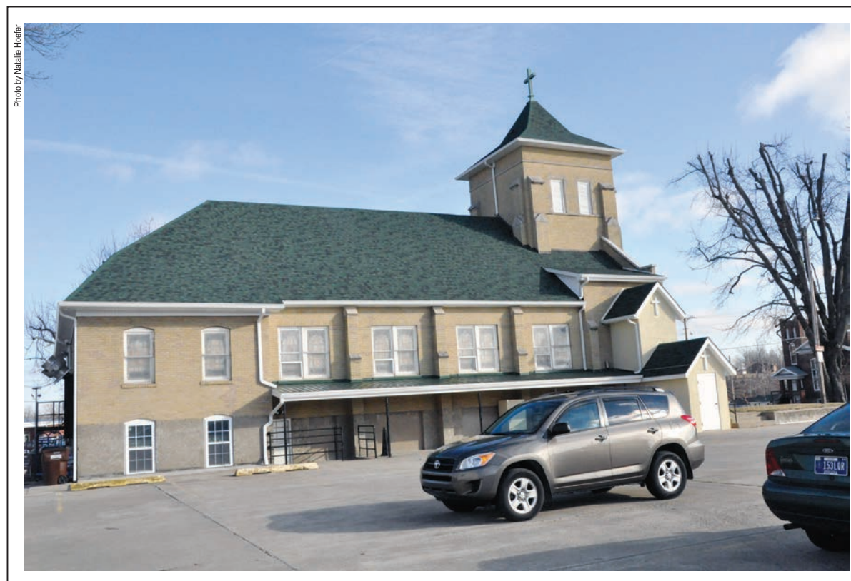
Above, St. Francis Xavier Church, including its renovated roof, is pictured in late February.
