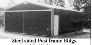
24'x40'x9' eave with (1) 12x8 end slider & (1) standard service door erected on your level site
