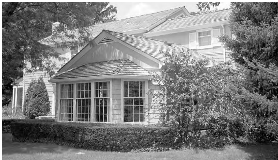
#1 Grade Red Cedar Shingle with Copper Flashing
